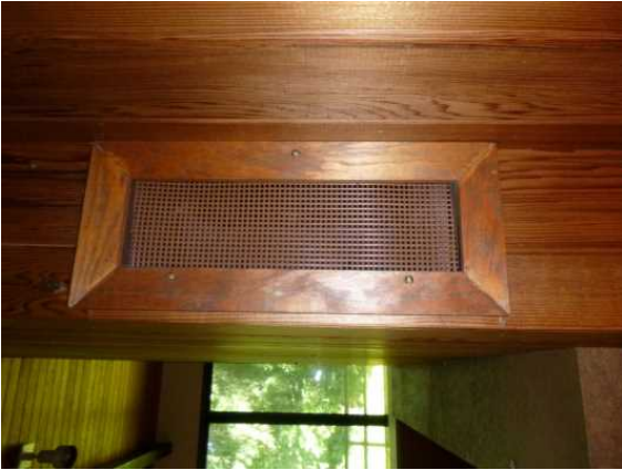
28 - Detail of original wood fireplace vent
