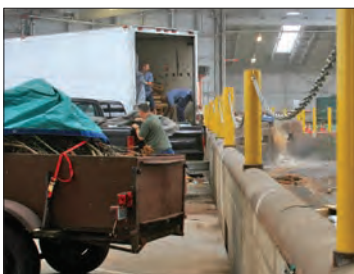
Customers unload waste onto the receiving floor
