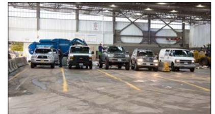
New transfer building has large self-haul customer unloading areas
