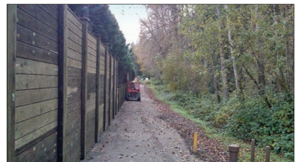
Constructed in 2011, a sound barrier wall along the west side of the transfer station helps reduce noise impact to neighbors
