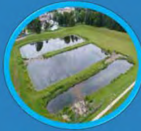
Storm water management
