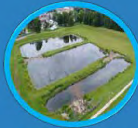
Storm water management
