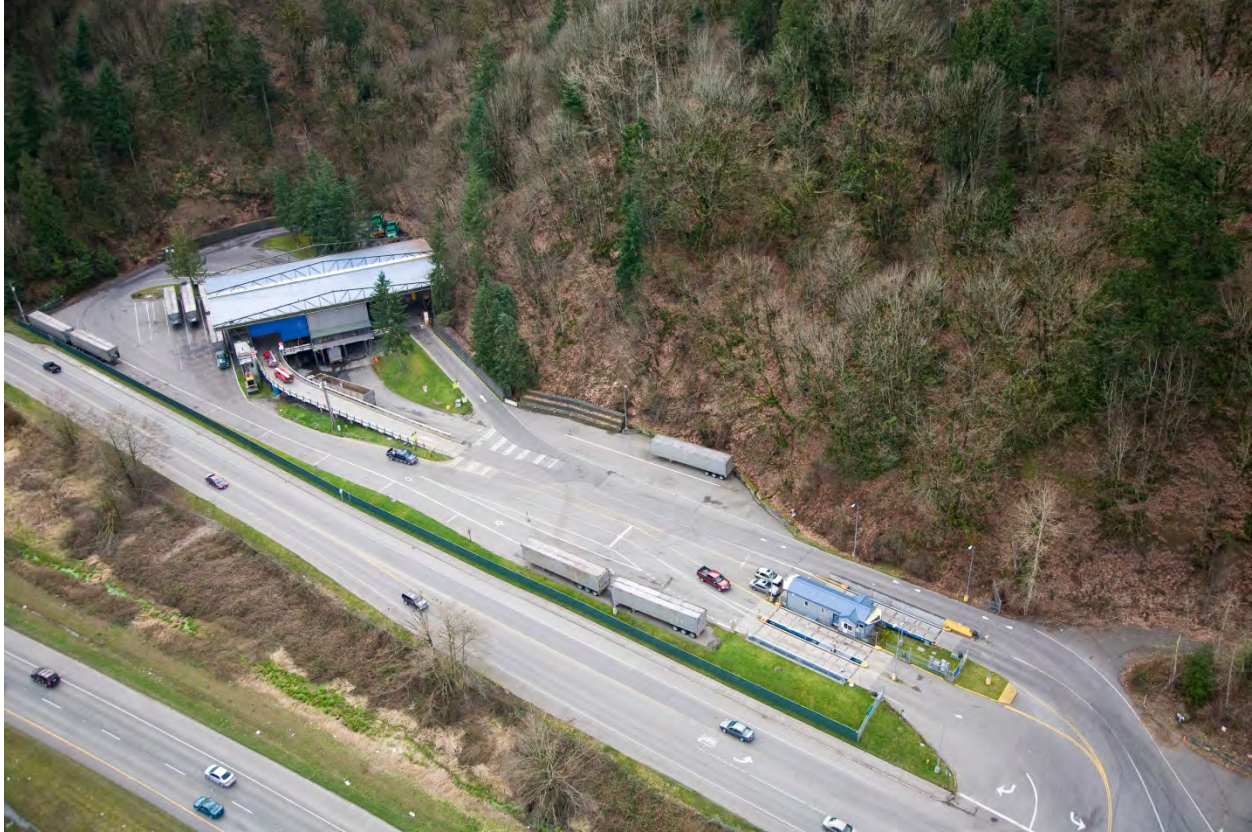
Figure 2-2: Aerial View of Existing Transfer Station
