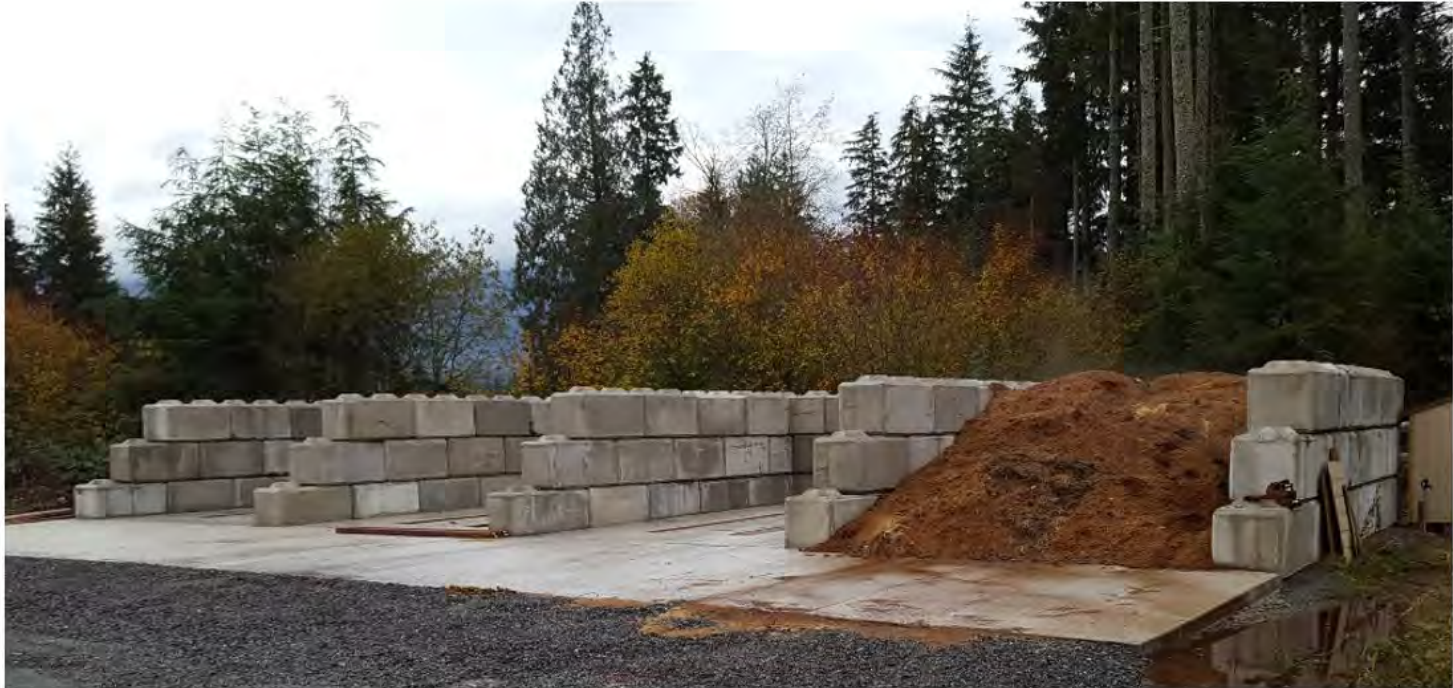
Aerated static pile in-floor positive system used in Sultan, Washington. Photo courtesy of O2Compost.
