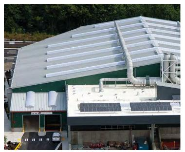
Solar panels and skylights on the roof of the new Bow Lake station are reducing resource consumption at the facility.
