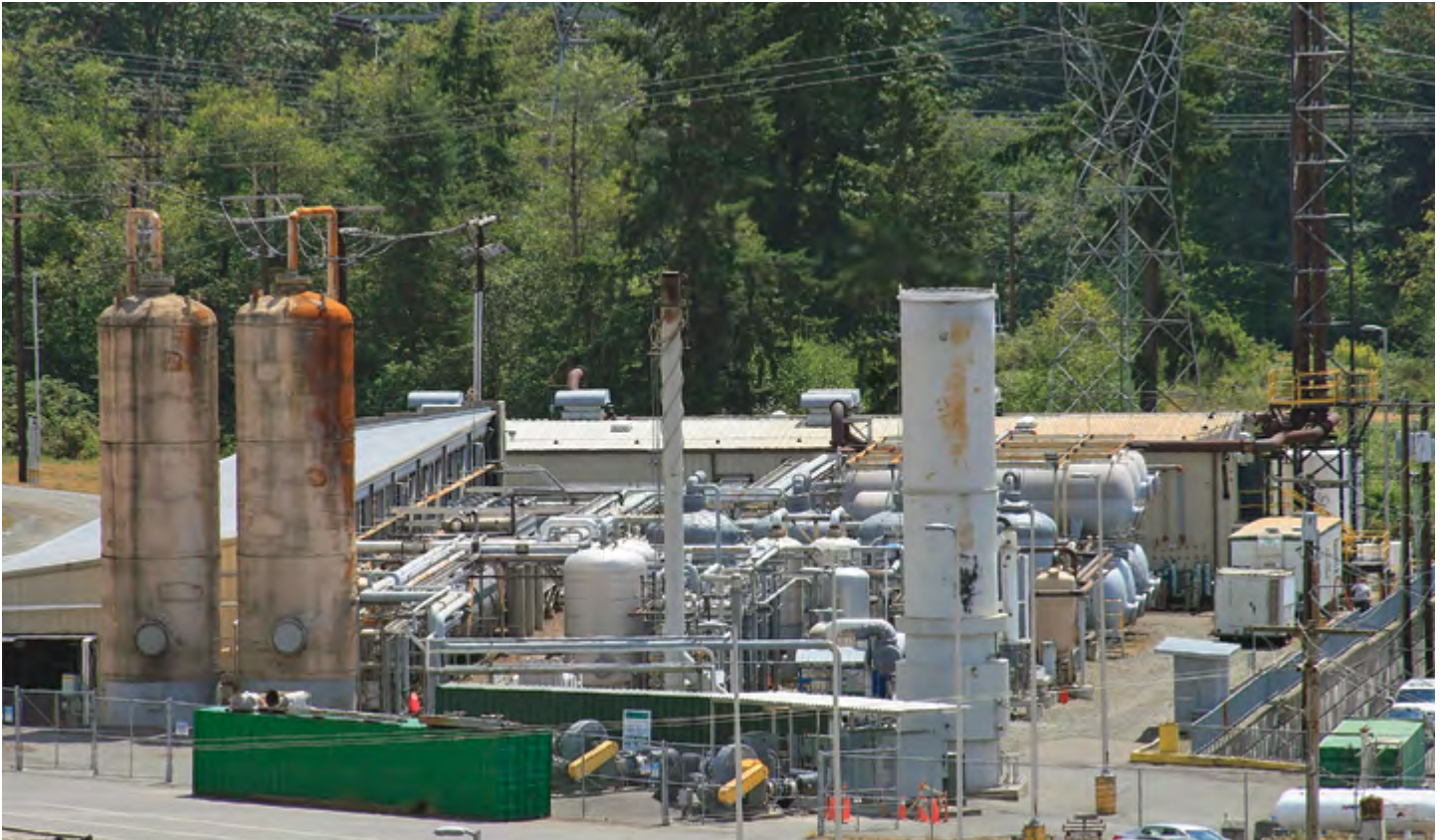
The onsite Bio Energy Washington facility processes landfill gas into a renewable energy source
