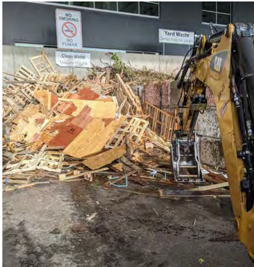
Figure 16. Usage of Machinery to Create Wood Pile, Resulting in Mixing and Breakage
