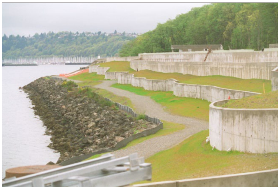
Figure 14. Walls Around West Point WWTP After Construction in 1995. Photo: King County.
