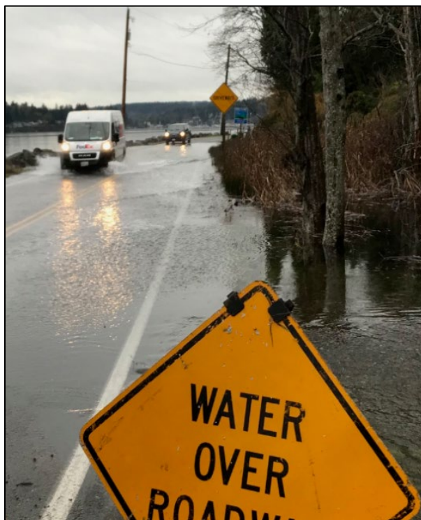
Figure 7. High Tide During a Storm Event (January 04, 2021). Overtopping of Quartermaster Drive and Inundation of Adjacent Property. Photo: KC Staff (G. Rabourn)
