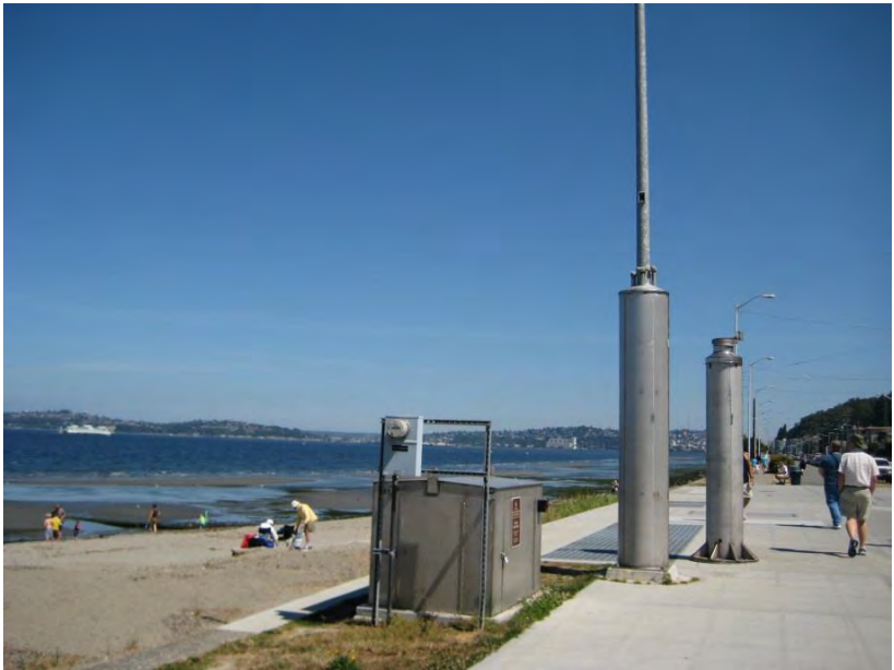
View of the exhaust stacks, electrical vault and public walkway on top of the pump station.
