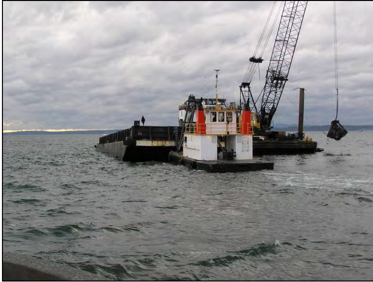
Figure 5-3. Dredging of Contaminated Sediments at the Old Denny Way CSO Site
