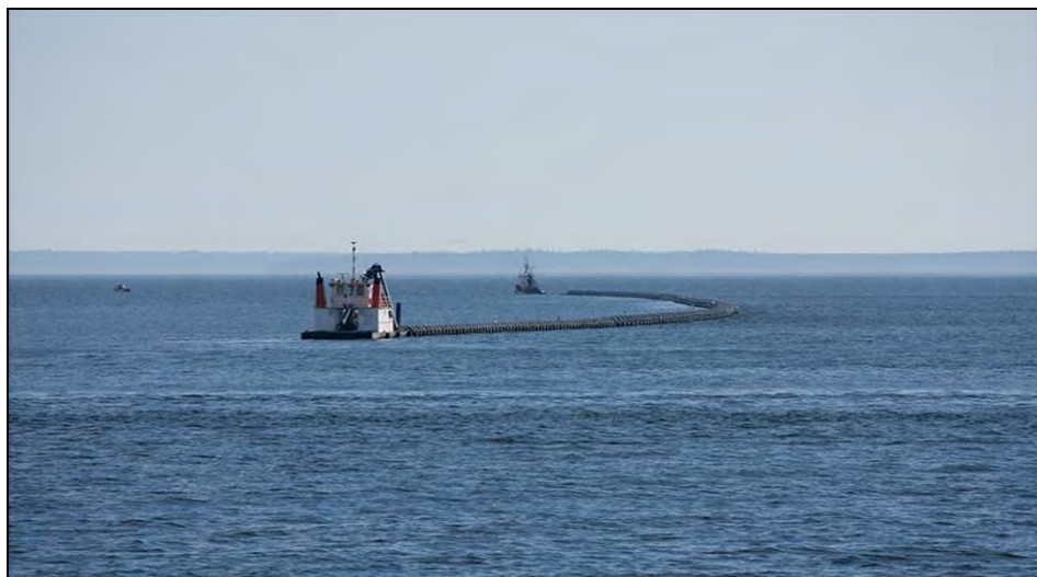
Figure 2-6. Towing of the Outfall Pipes
