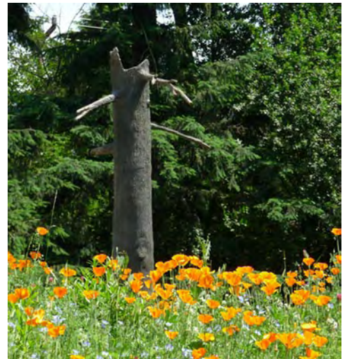
Hidden Lake Sewer Improvement Project - odor control stack disguised as a tree snag in Boeing Creek Park
