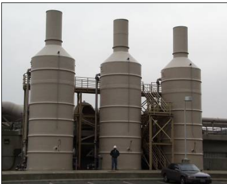
Figure 2-1. Primary Process Odor Scrubbers at West Point Treatment Plant
