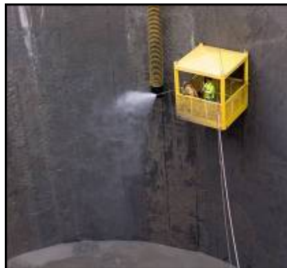
Workers cleaning the walls of the Influent Structure Shaft
