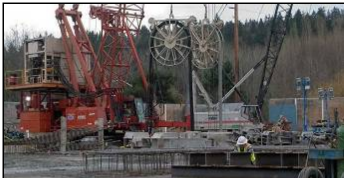
Workers use a hydromill trench cutter to excavate the slurry walls for the Influent Pump Station
