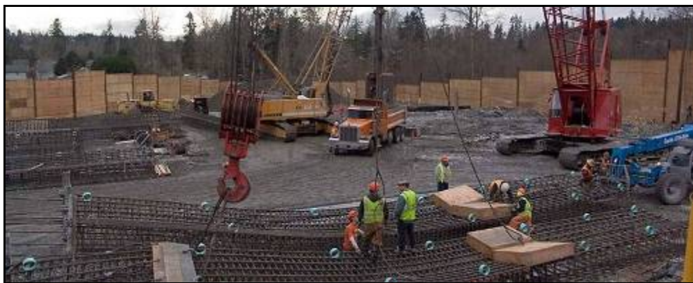
Workers construct rebar cages for the slurry walls at the North Kenmore Portal site
