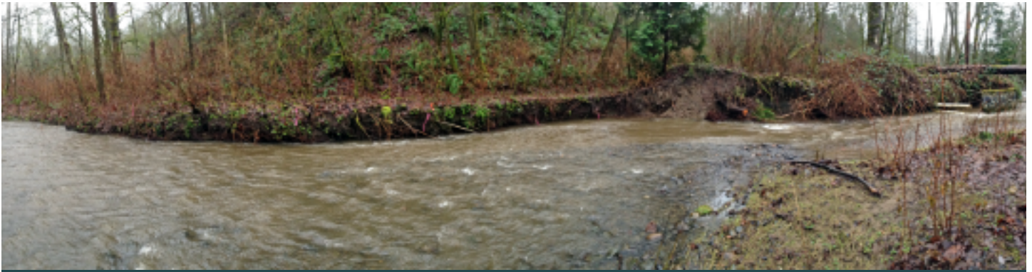
Creek flooding has eroded the bank that protects the Coal Creek sewer pipe
