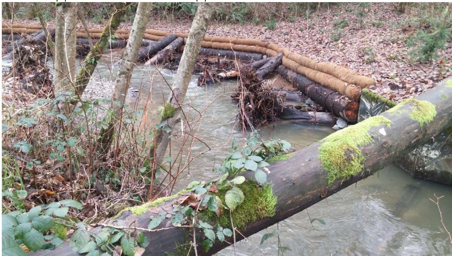
After a large flood, WTD carried out extensive bank repairs to protect the sewer pipe.
