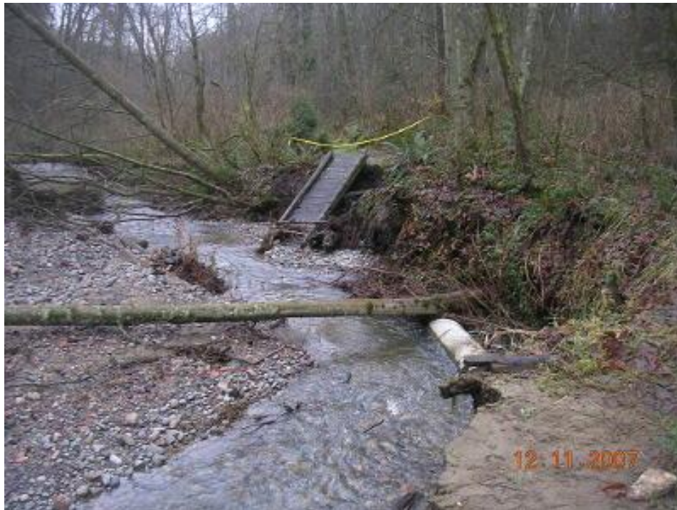
This image shows the Coal Creek after a major storm in December 2007. The creek scoured the bank, exposing the pipe, visible underneath the fallen tree.
