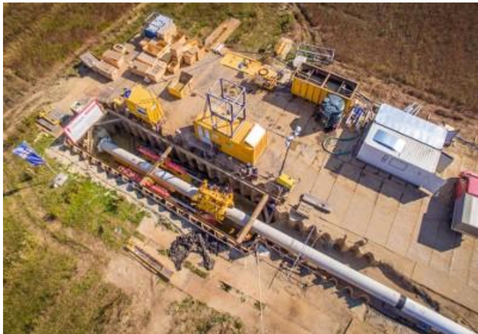
Image of launch pit from Herrenknecht.
