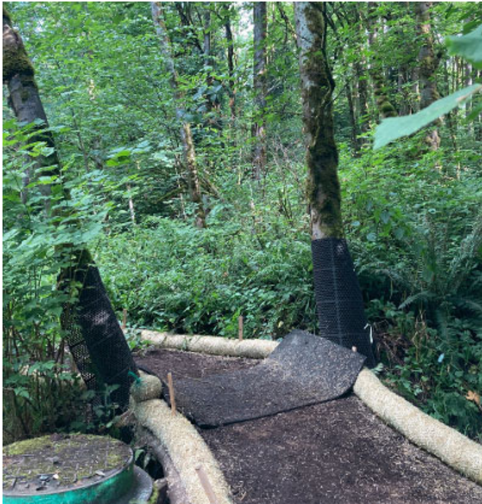
Fabric logs, mats, and guards protect the roots and bark of trees along a trail in a work area.
