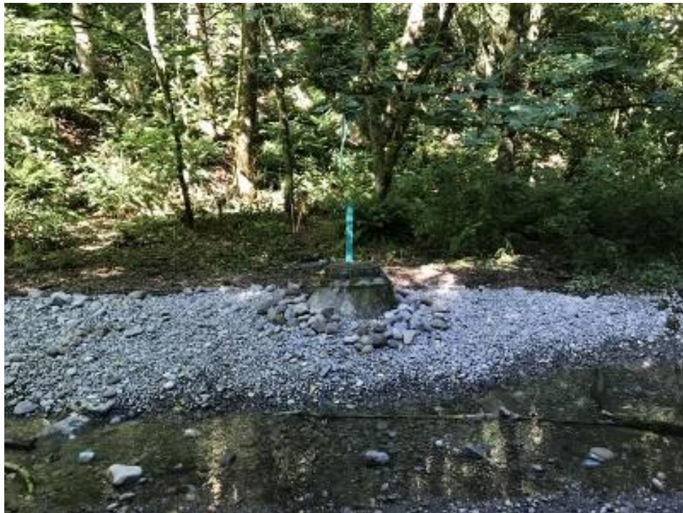
A temporary maintenance hole protection project was completed in August 2020. This structure will be removed as part of the project.
