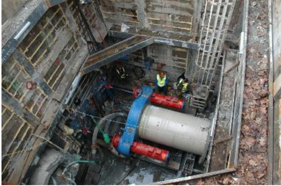
This photo shows a typical microtunneling entry pit.
