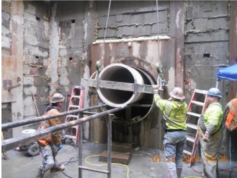
This photograph shows an outer casing pipe and a smaller white pipe inside the casing.
