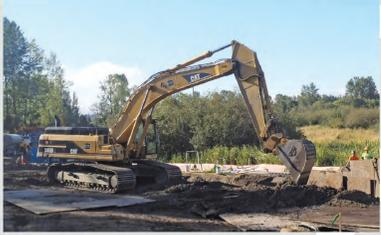
**1.** The contractor will use open trench methods to connect the new Coal Creek pipe to the East Side Interceptor that carries to South Treatment Plant. Landscape restoration will follow.
