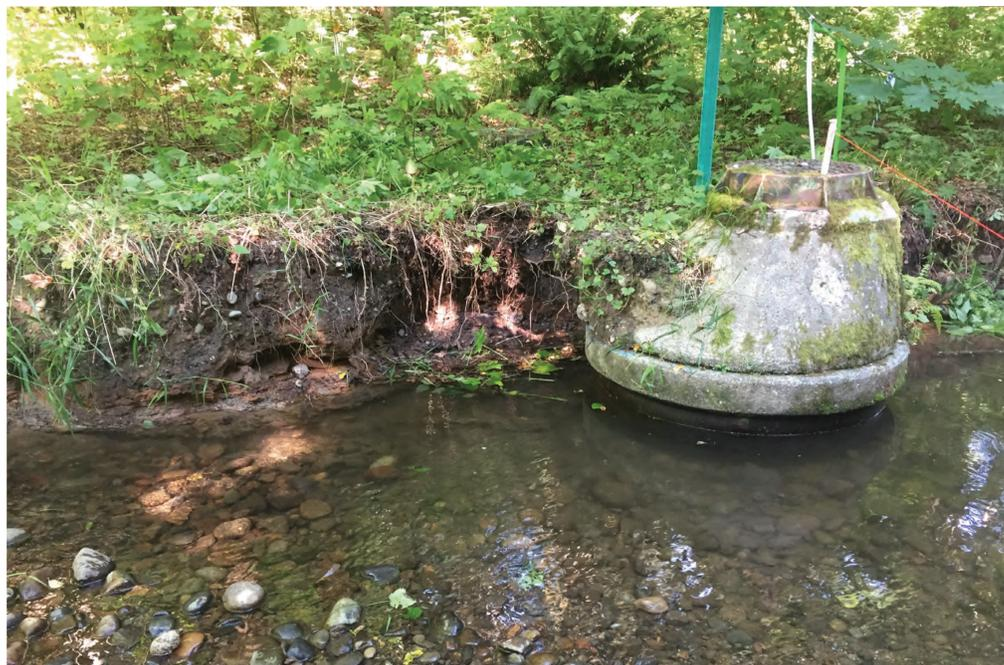
Flooding in December 2019 eroded the bank around this maintenance hole (left). A temporary repair project (right) will help protect the structure until the project is completed in 2027.
