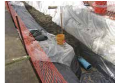
Installing drain pipe
