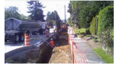
Digging out the planter strip
