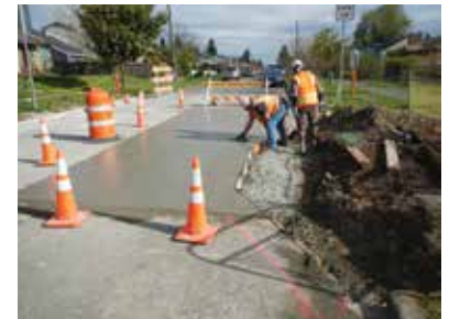
Replacing street panel with new curb bulb in place
