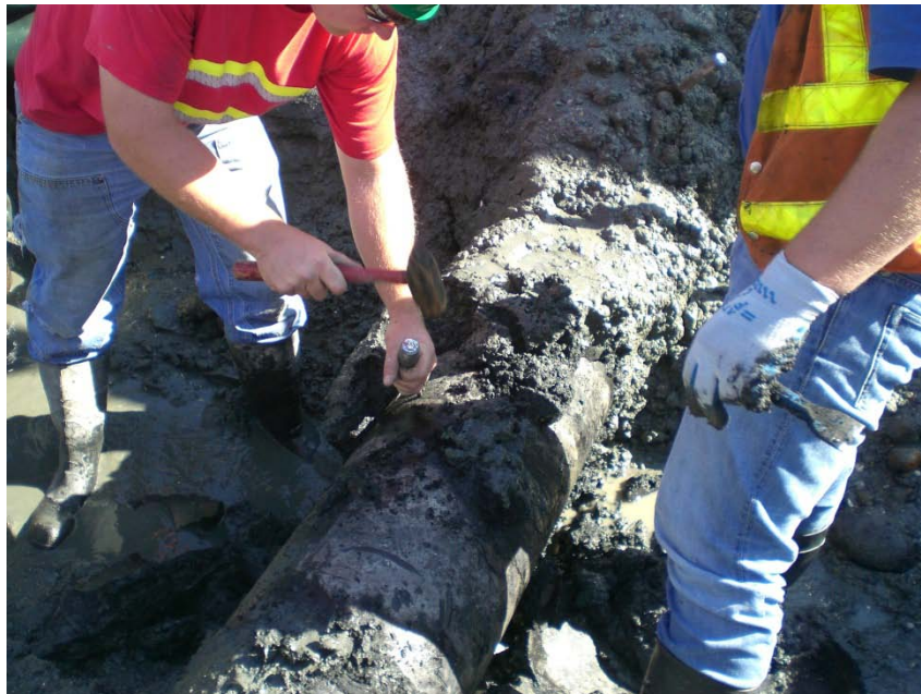
Picture 3-2: Pipe Surface Visible while Tapping Crew Removes Carbonation Layer
