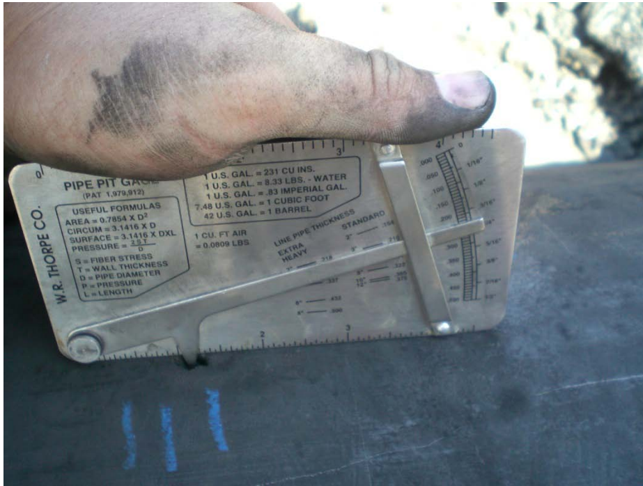
Picture 3-5: Depth of Pit 3
