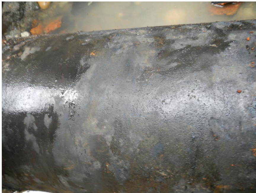
Picture 1-6: Profile Cleaned Cast Iron
