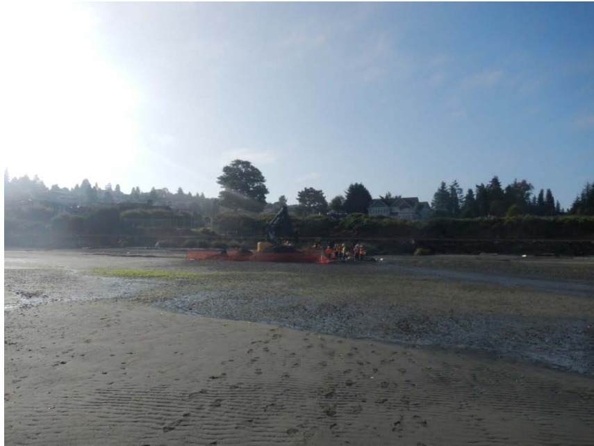
Picture 1-1: General Overview of Excavation
