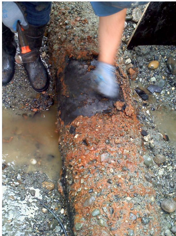
Picture 1-4: Carbonation Layer Removed to Bare Pipe Surface
