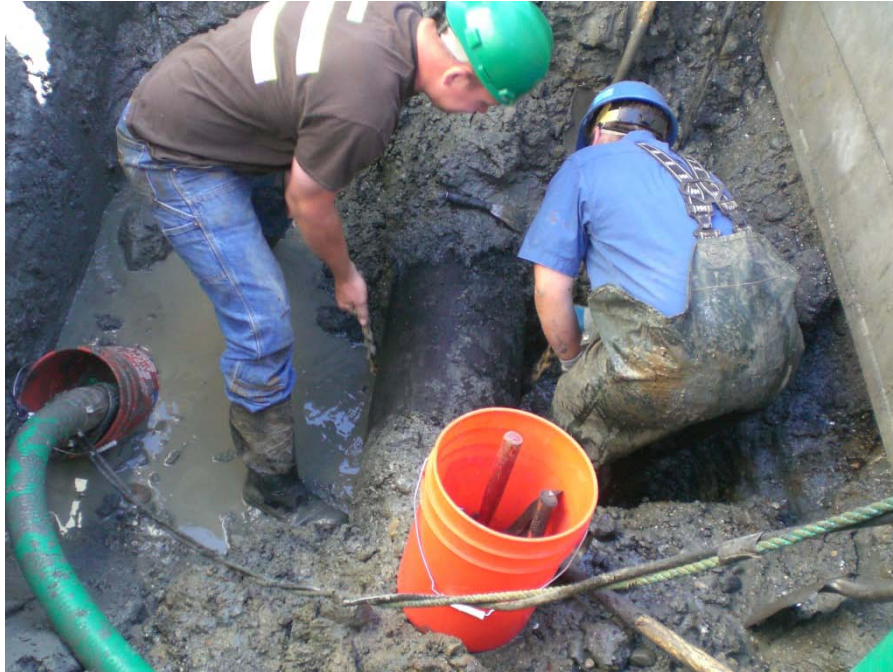
Picture 2-3: Carbonation/Corrosion Layer Being Removed by Tapping Crew
