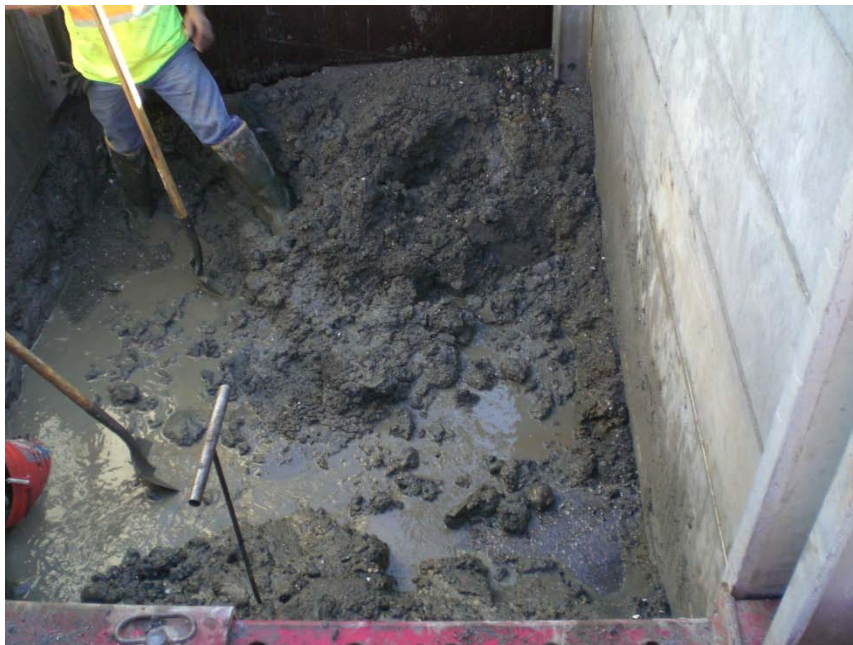
Picture 2-2: General Soil Conditions Surrounding Pipe
