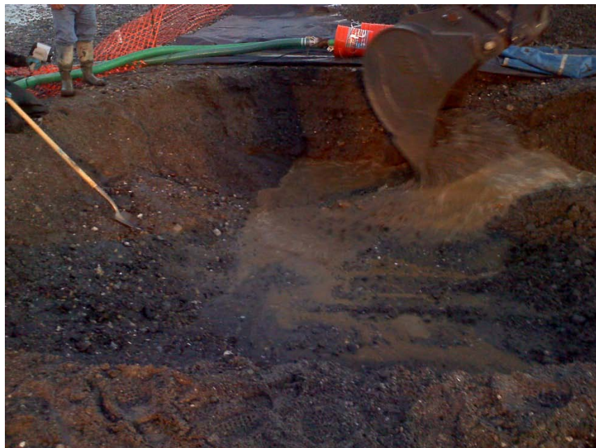
Picture 1-2: Excavation at Beginning Stages Depicting Water Level
