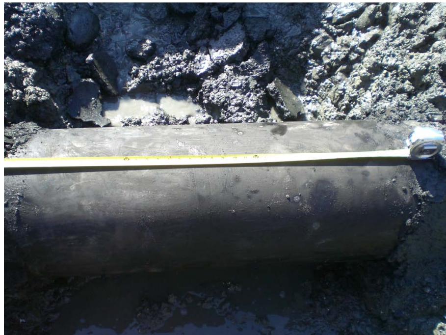
Picture 3-4: General Profile of Cleaned Pipe
