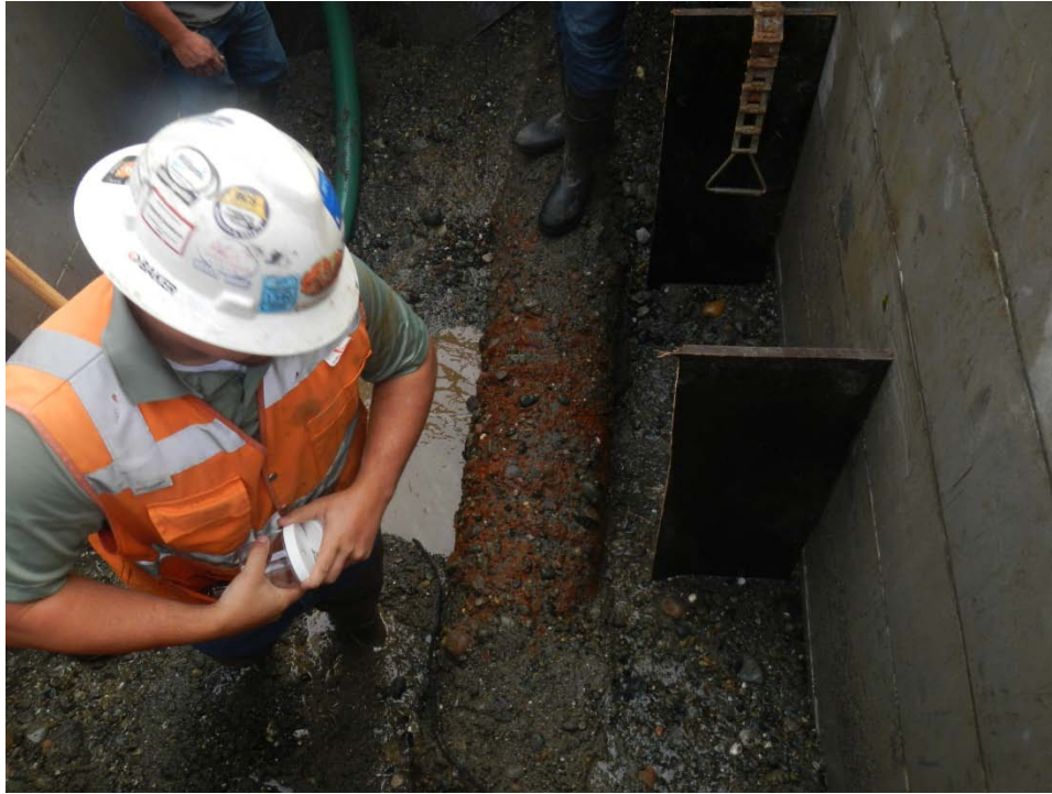
Picture 1-3: Pipe with Carbonation Layer Intact
