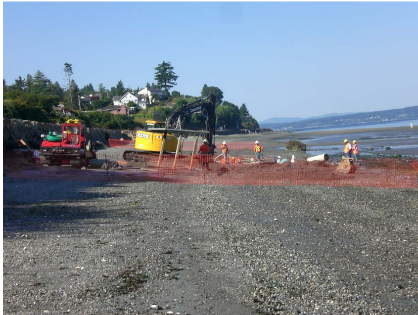
Picture 3-1: General Overview of Excavation
