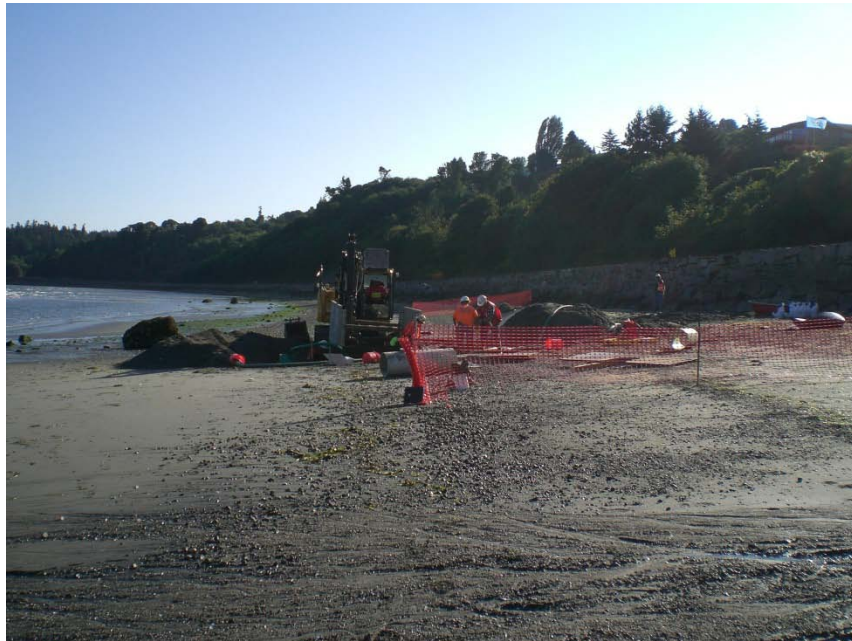
Picture 2-1: General Overview of Excavation
