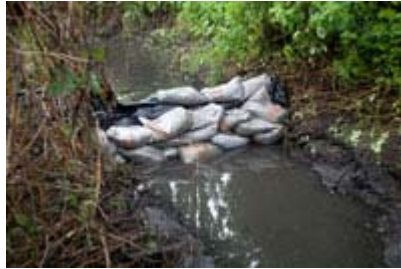
Dams were built to contain the cleanup area. June 6, 2008
