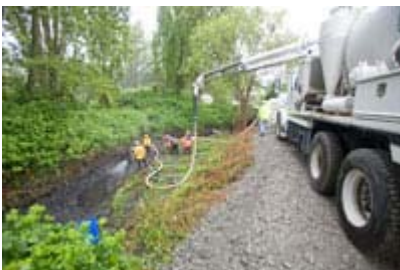
Vactor trucks supplied water to wash sediment from banks and the bottom; the resulting slurry is drawn up into the vactor truck. June 6, 2008
