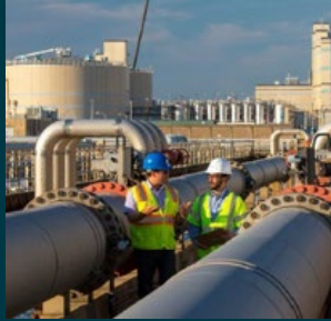
Biosolids, Energy Recovery and Optimization
