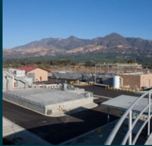
Wastewater Treatment, Recovery and Reuse
