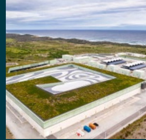
Advanced Treatment and Desalination
