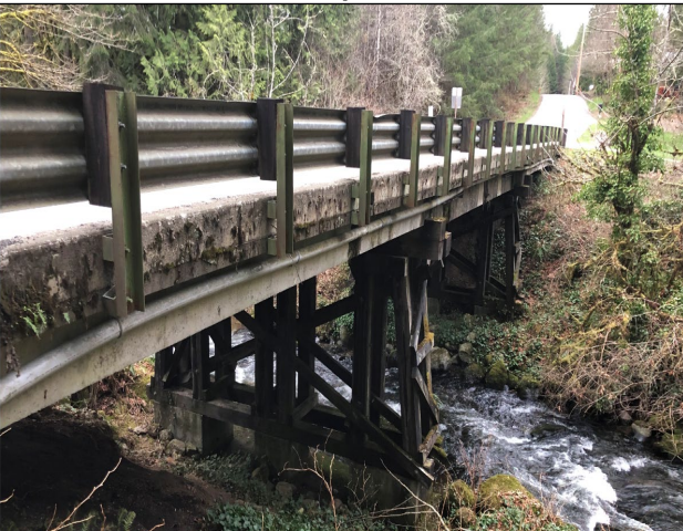
Upper Tokul Creek Bridge 271B Prior to Replacement
