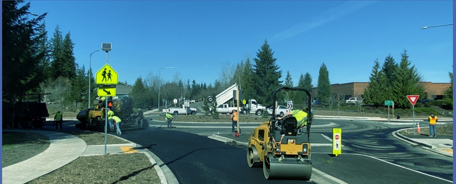
Redmond Ridge Roundabout
