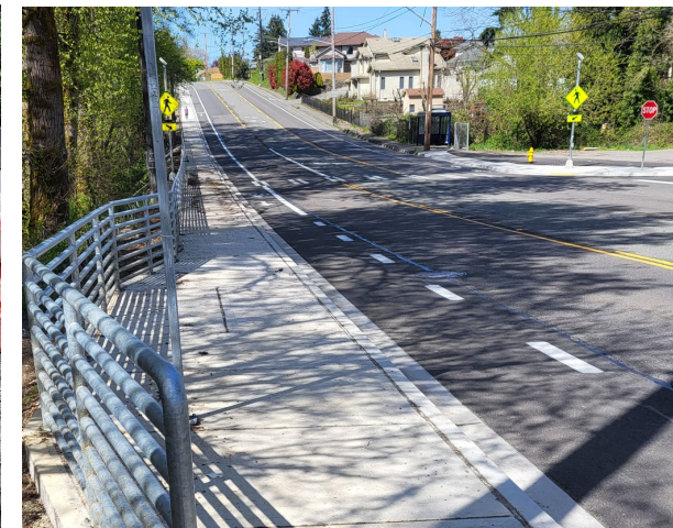
Renton Ave S Sidewalk, Phase III
