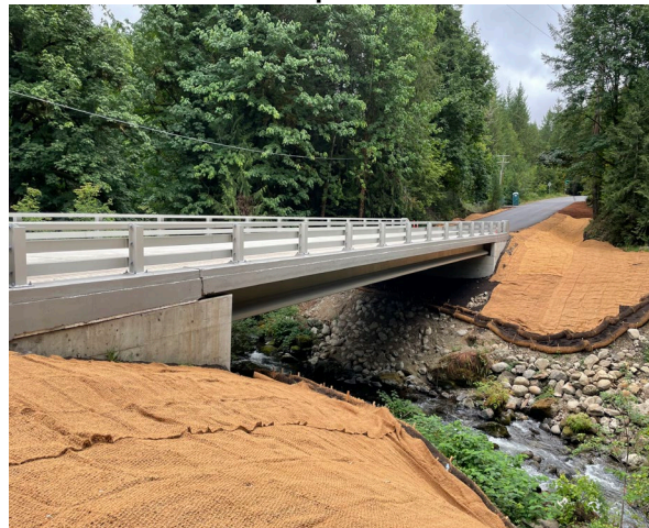
Upper Tokul Creek Bridge 271B After Replacement
