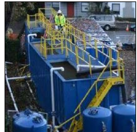
Dewatering equipment will stay in place until foundations are removed.
