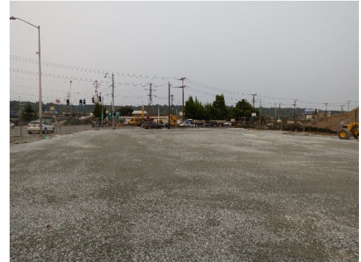
Site preparation and demolition is complete
