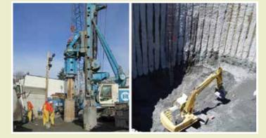
Secant pile installation is expected to be complete by this fall. A video showing an example of secant pile wall construction is available on our website.
