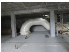
Once wastewater is treated through the ballasted sedimentation process, it will flow to the UV disinfectant tanks through this effluent pipe.
