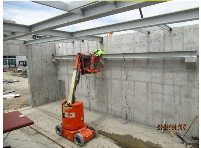
Steel work at the treatment station's operations and maintenance building.
