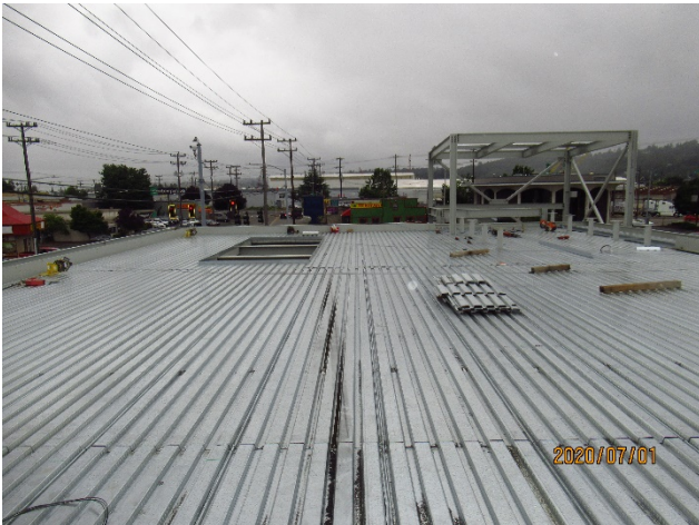
Pan decking on the operations and maintenance building on the treatment station site
