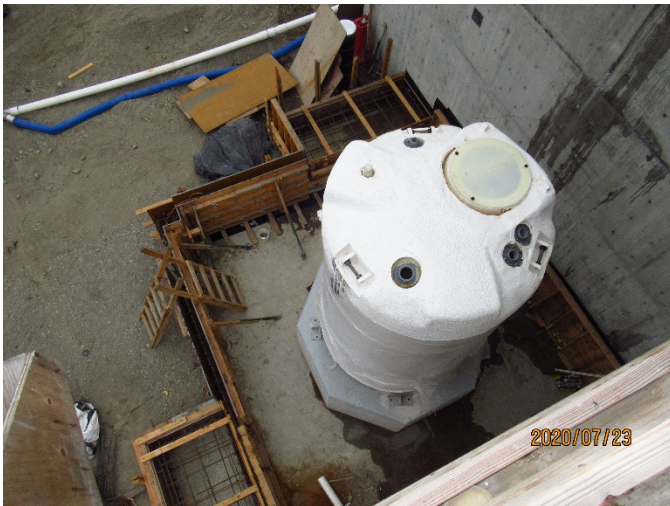
A coagulant tank is installed at the treatment station site
