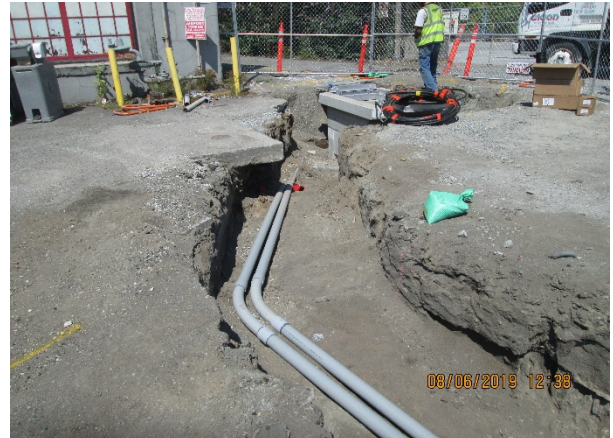
Temporary electrical connections
