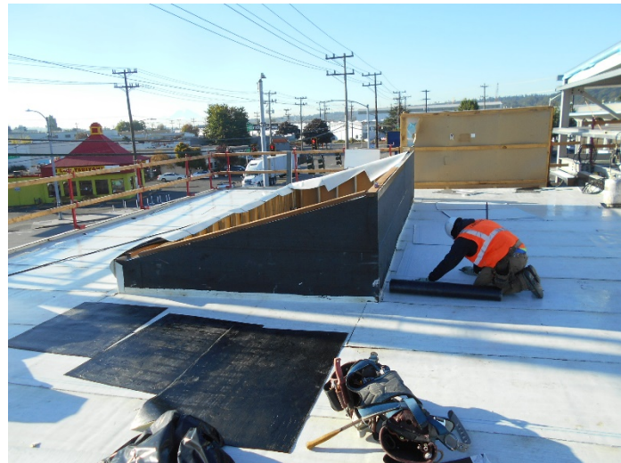
A skylight installed at treatment station's operations building
