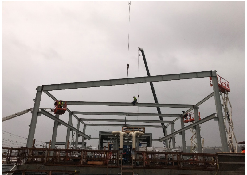
Steel frames are erected at the Ballasted Sedimentation building
