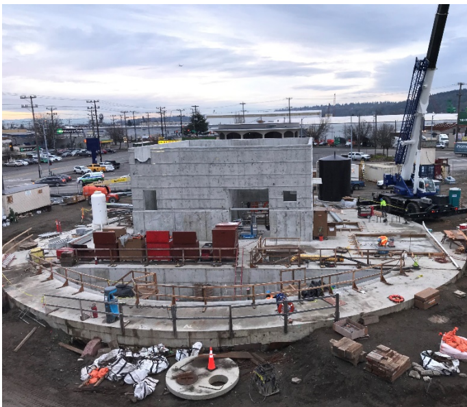
An aerial view of the equalization basin
