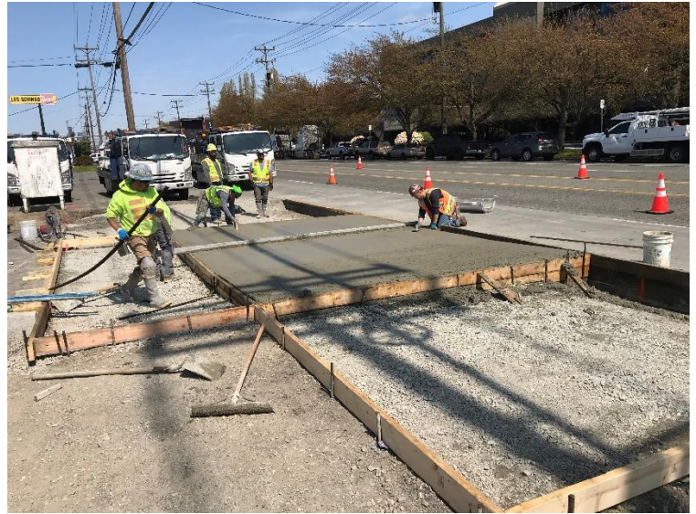
Crews form and pour new concrete on 4th Avenue South.
