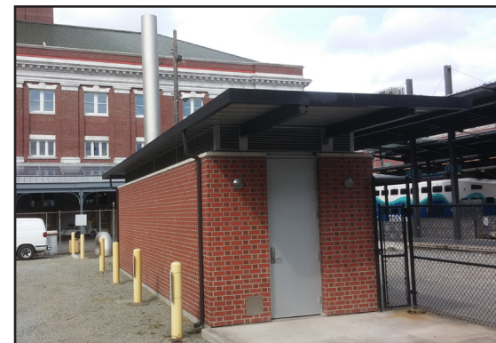
Example of a building that houses equipment to support the carbon scrubbers.
