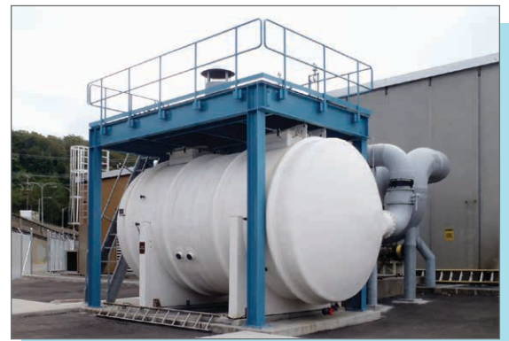
Carbon scrubber at Interbay Pump Station
