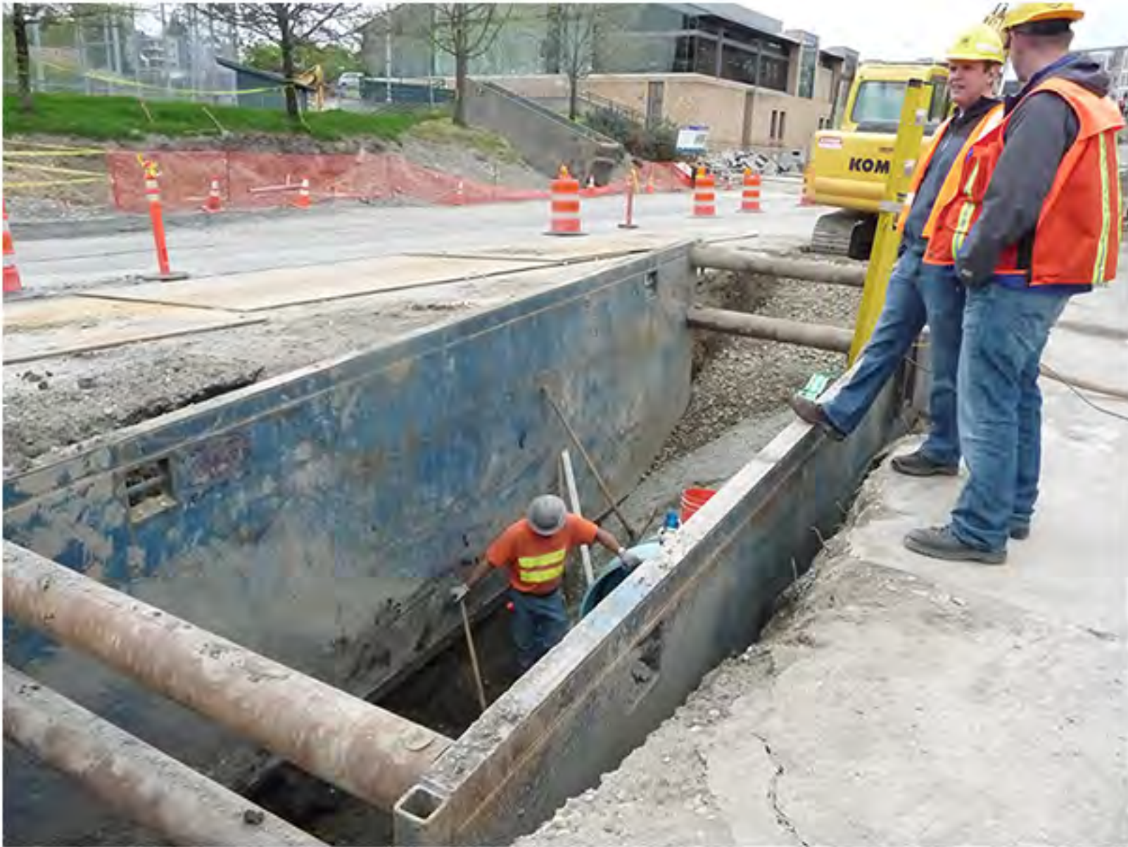
Open-trench construction will be used to install the majority of the pipe.
