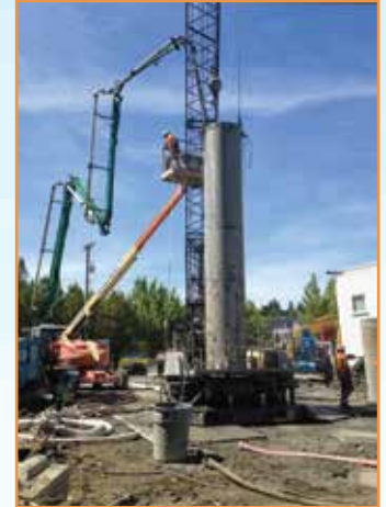
Shaft construction using interlocking concrete cylinders.
