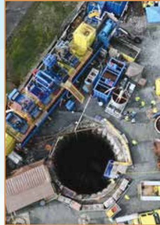
Shaft construction using interlocking concrete cylinders.
