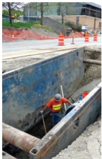
An example of open-trench construction.
