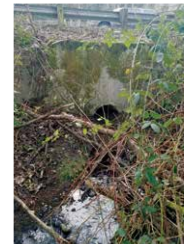
Existing culvert at Country Creek
