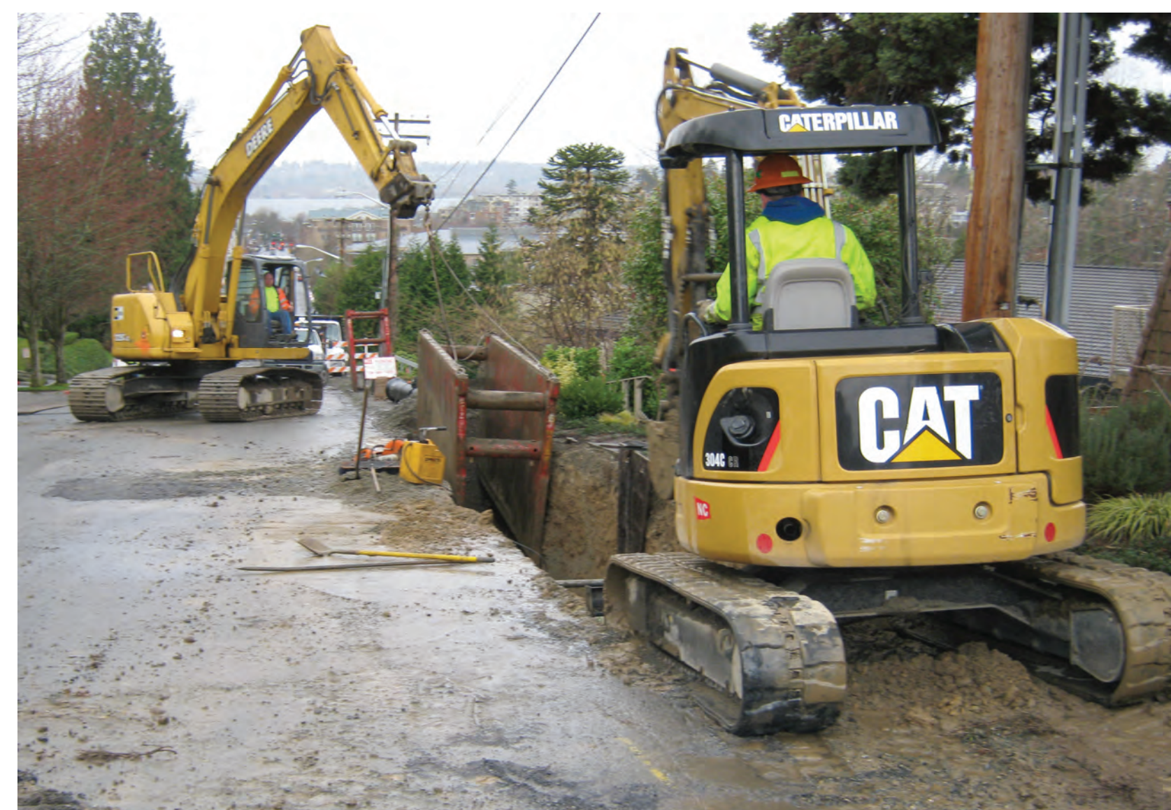
Crews excavate before open-cut installation
