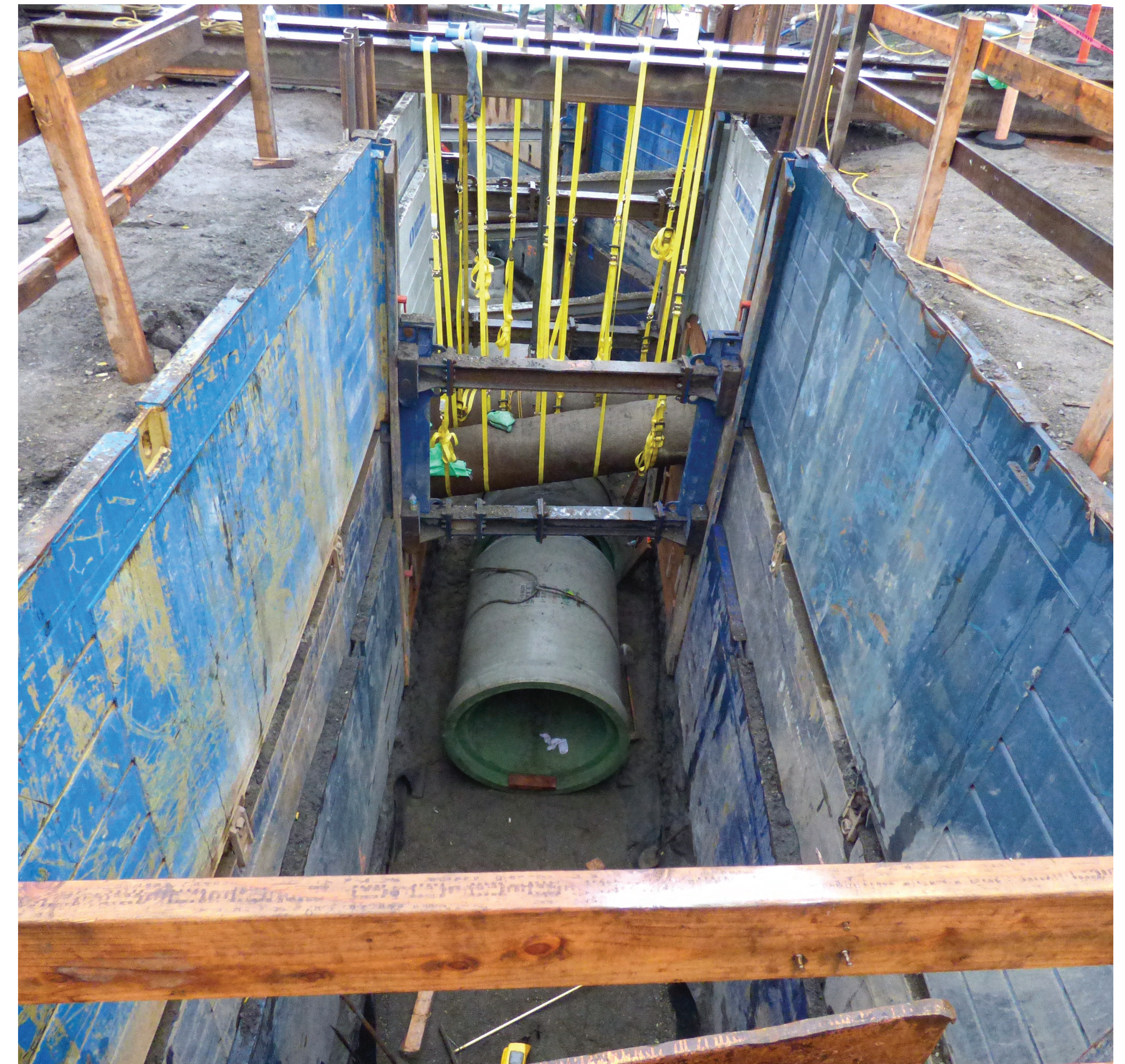
Example of open-cut installation of 60" pipe
