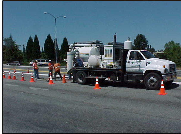
Typical vacuum truck used for potholing work.
