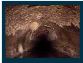
The M Street Trunk is deteriorating and needs to be rehabilitated so the pipeline does not fail, overflow, or disrupt sewer service resulting to impacts to public health and the environment.
