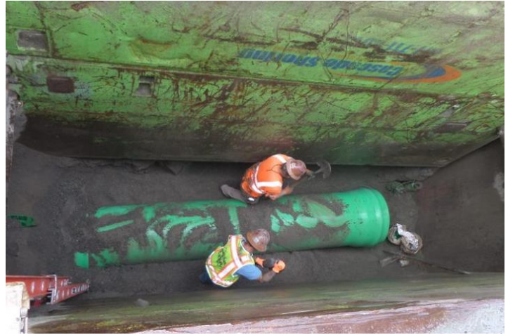
Crews install pipe deep underground via "open cut" construction.
