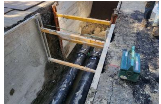
Crews install pipe under the right-of-way on 90th PI S.E.
