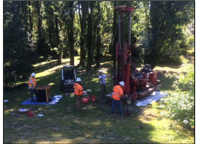
Typical drill rig.
