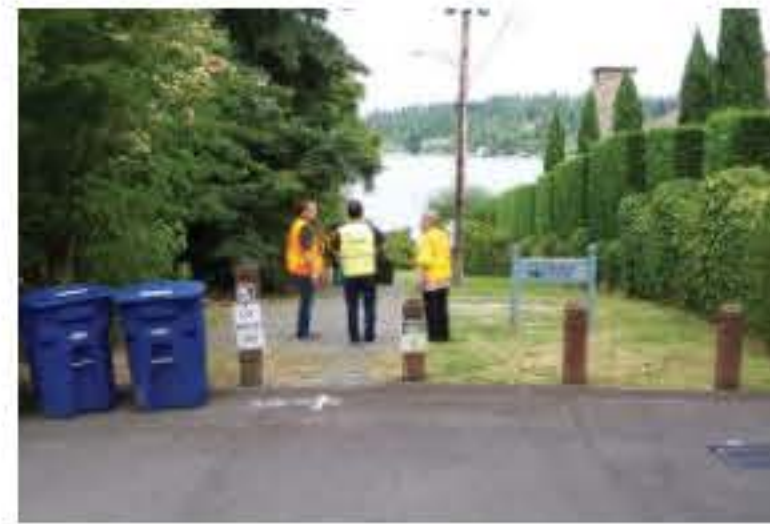
Lift Station 11 at Fruitland Landing
