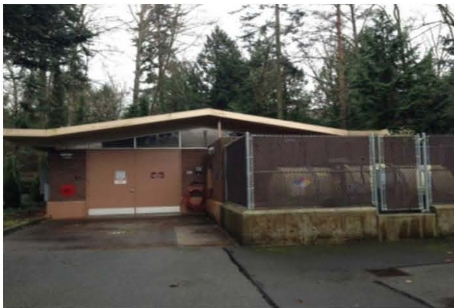
Existing North Mercer Pump Station, 7631 SE 22nd St, Mercer Island
