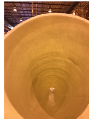
Step 4: Completed New Structural Pipeline
