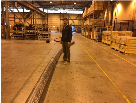
Step 1: Insert Liner in Pipe And Inflate Liner
