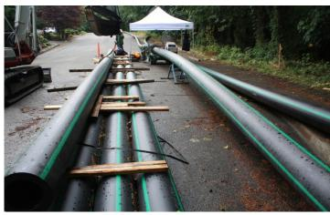
While the drilling crew is preparing the bore hole, a crew uses heat to fuse pipe sections together. The growing pipeline is laid out in long strings. On the day of pullback, the strings are fused together and pulled through the borehole.
