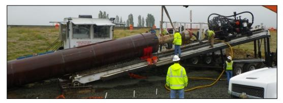
To protect the surface, crews will install steel conductor casings underground prior to drilling the pilot bore.
