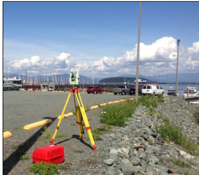
Crews will use total stations and other handheld equipment to take survey readings.
